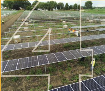
Solar module installation then gets underway! Each module has a generating capacity of 340-445 watts.
