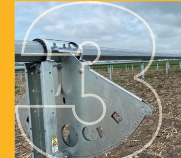
Bearing housings sit on top of the piles to support movement from torque tubes. The torque tubes connect and form a row, holding the racking that houses the solar modules.
