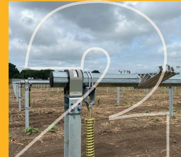
Motors are attached to drivelines, which are then used to rotate rows of torque tubes topped with solar modules. This allows the solar modules to track the sun from east to west to ensure maximum electricity generation.
